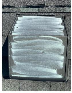
Accessory - Back - 1st Story Slope Box Vent Aluminum Storm related damage caused by hail June 1, 2023
