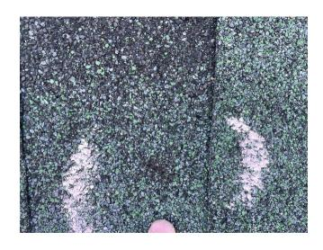
**Left - 1st Story Slope - Damage** Storm Related Damage caused by Hail June 1, 2023
