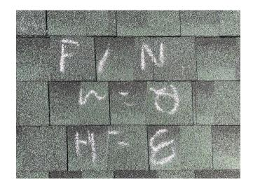
**Front - 1st Story Slope - Damage** Storm Related Damage caused by Hail June 1, 2023
