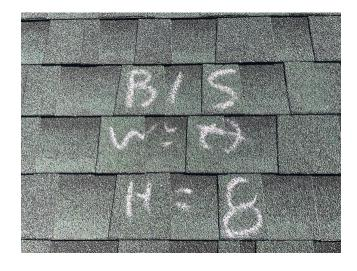
**Back - 1st Story Slope - Damage** Storm Related Damage caused by Hail June 1, 2023
