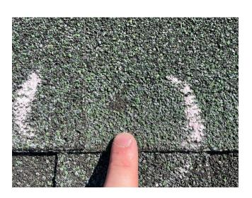
**Right - 1st Story Slope - Damage** Storm Related Damage caused by Hail June 1, 2023
