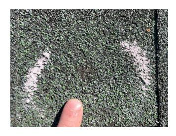
**Back - 1st Story Slope - Damage** Storm Related Damage caused by Hail June 1, 2023
